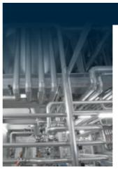
Welded stainless steel tubes according to EN 10217-7 TC1 or TC2 in austenitic grades: 4307 - 4404 - 4571 - 4541.
